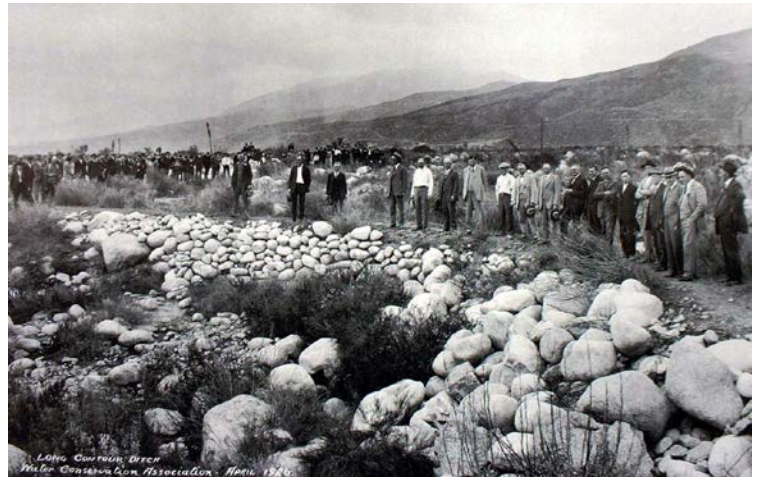
Contour ditch constructed by Water Conservation Association to conserve Santa Ana River water, Highland, Calif. April 1926
