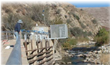
Cuttle Weir, off Greenspot Road
