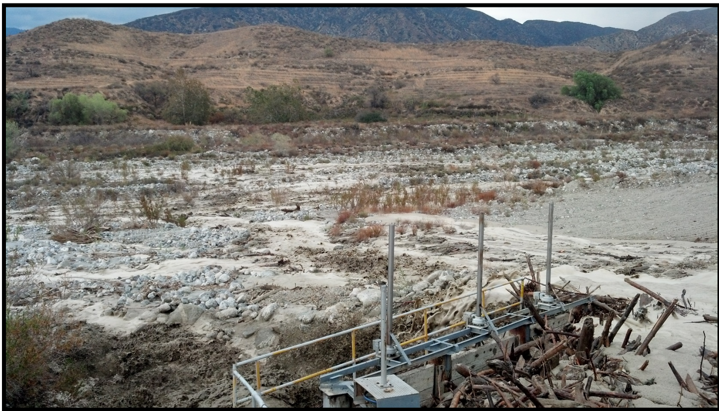
Photo 8 – Existing conditions of Debris Return Area during a typical high-flow event. Rip rap will be placed in this area for better debris flow and debris management.
