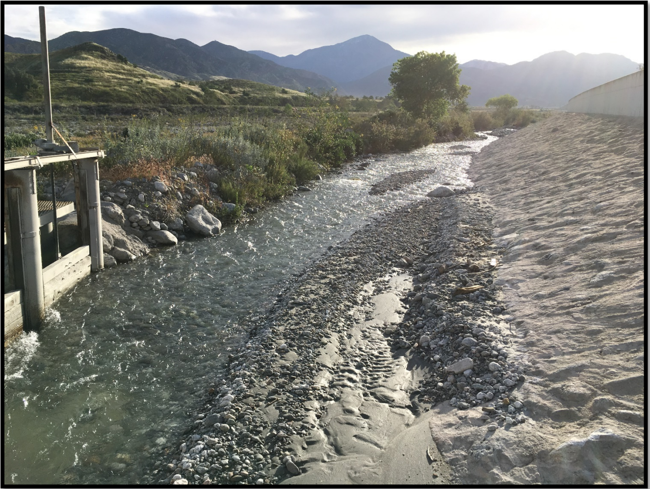
Photo 3 – Upstream of the Diversion Structure (Area of Work). Corps Levee consists of the concrete wall and the rip rap slope pictured on the right.
