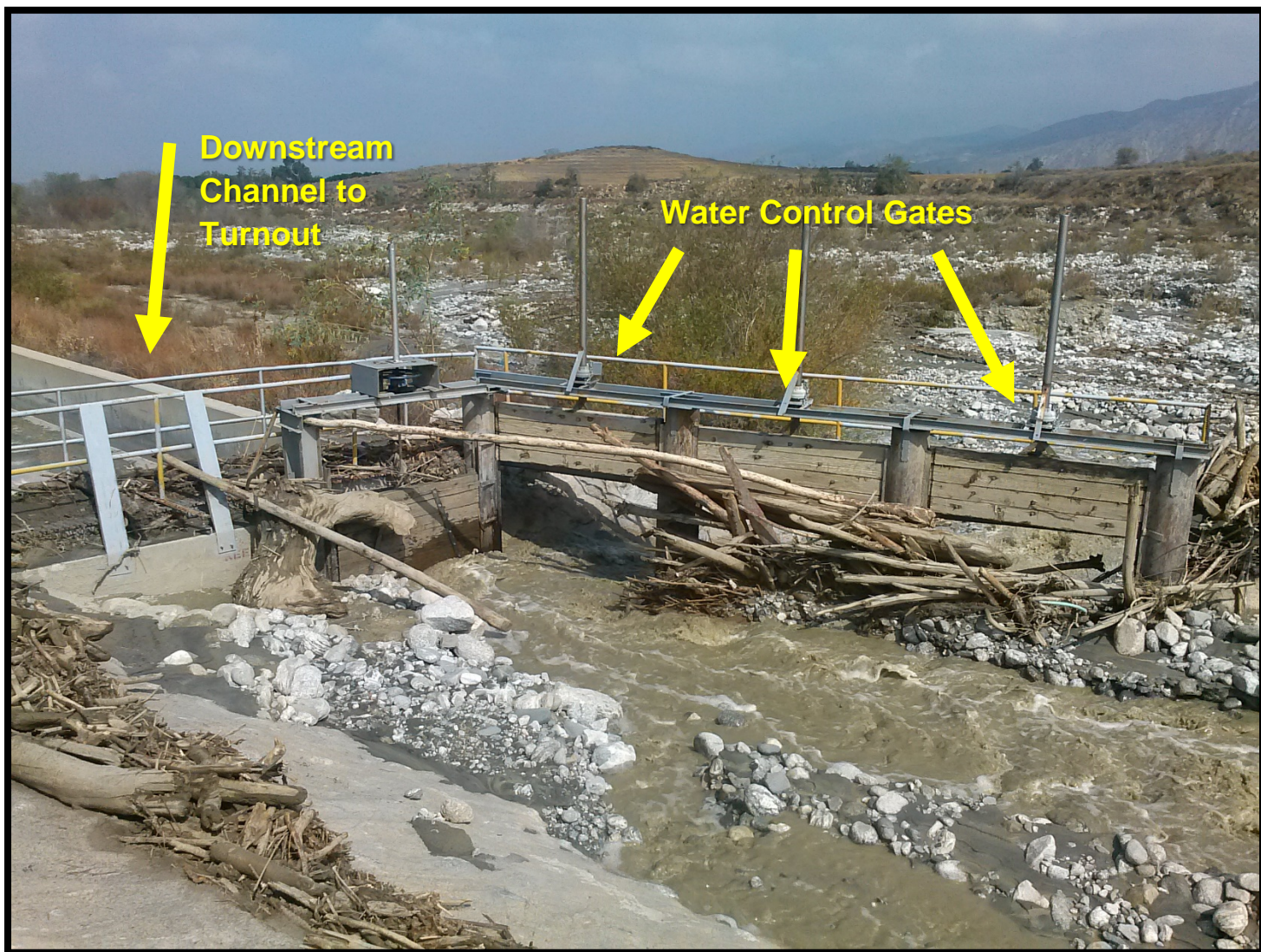
Photo 6 – Diversion Structure during a typical high-flow event. The wooden gates are lowered during normal operations to allow water to flow downstream to the turnout. The wooden gates are manually raised during storms to allow debris to return to Mill Creek. This demonstrates that the gates are undersized for a typical large event as the larger debris collects at the undersized gates. Photo also shows the location of the facility and the Corps levee slope.
