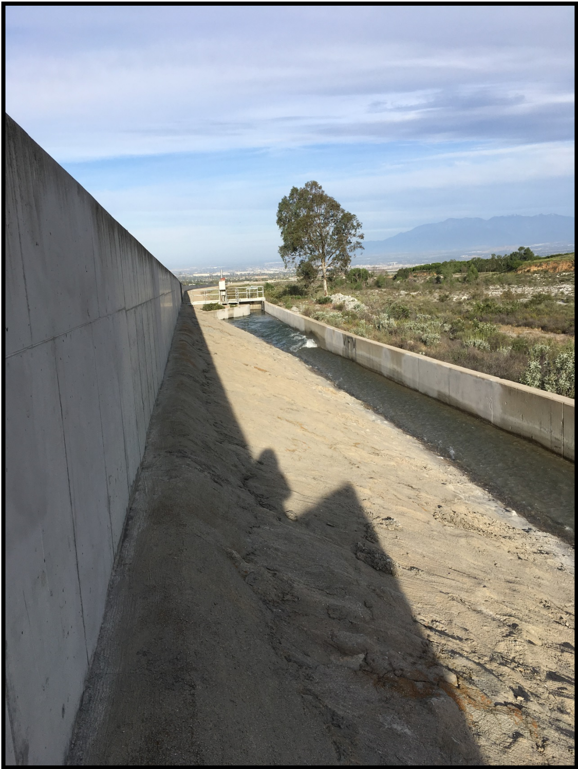
Photo 2 – Downstream of Diversion Structure. Corps constructed levee consists of the concrete wall on left and the slope. The Diversion channel concrete wall is pictured to the right of the channel. Photo depicts the water channel downstream of the Diversion Structure, where the final flows are directed from the Structure to the turnout that leads to the water conservation basin south of the levee.
