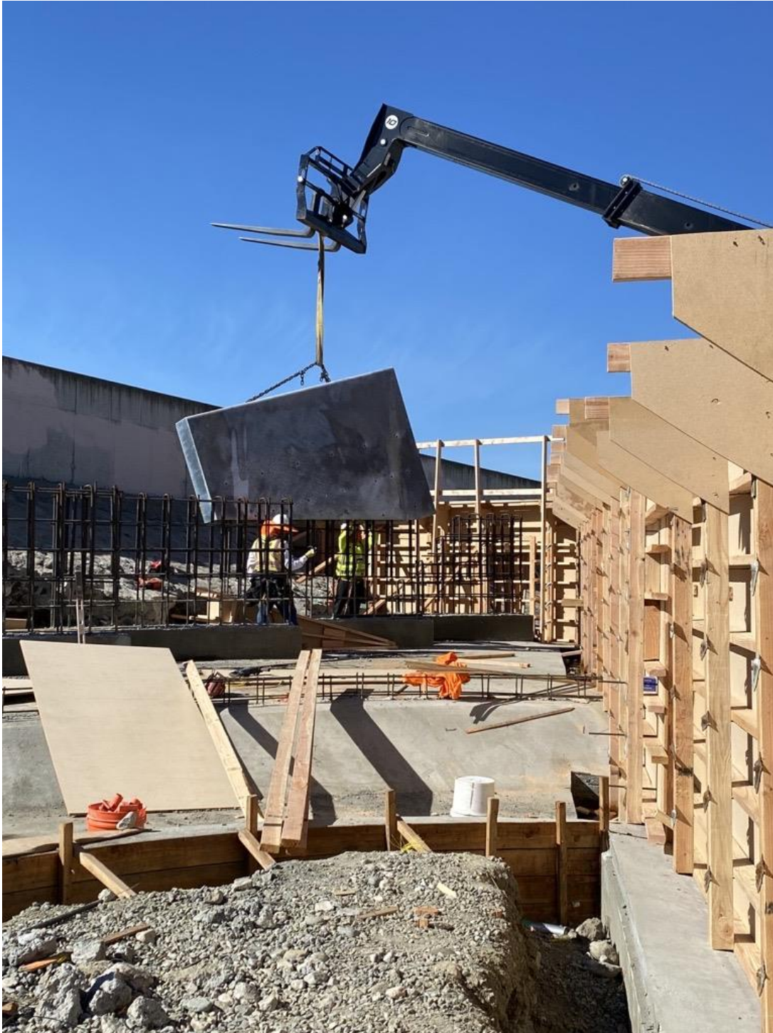
Placement of 1-ton Hollow Steel Diverter Walls at the Mill Creek Diversion Project
