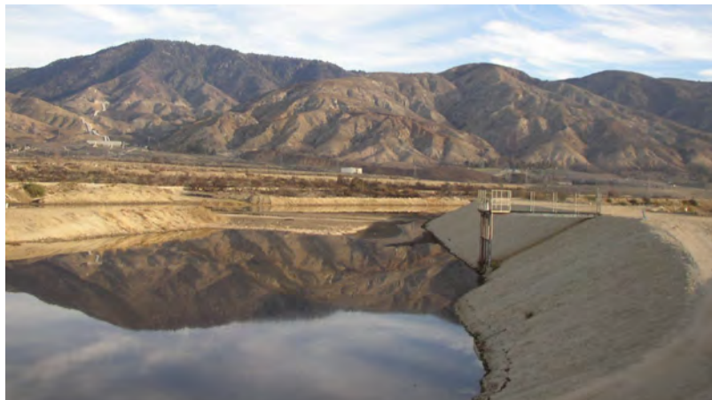
Numerous groundwater spreading grounds have been developed to recharge the groundwater basins.
