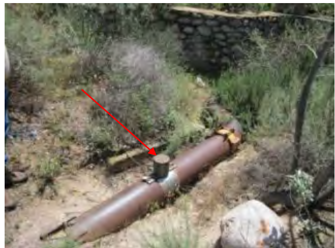
There is a flow meter locked inside a steel cover (red arrow).
