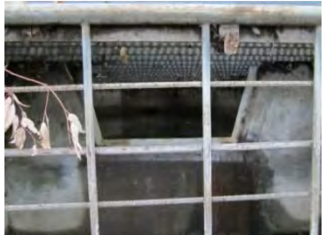
Inside of structure, weir can be used as backup measurement.
