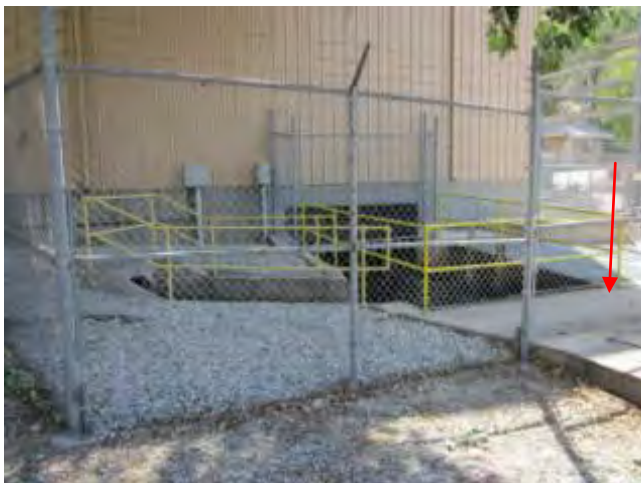
Excess water exits the Afterbay through weir (red arrow).
