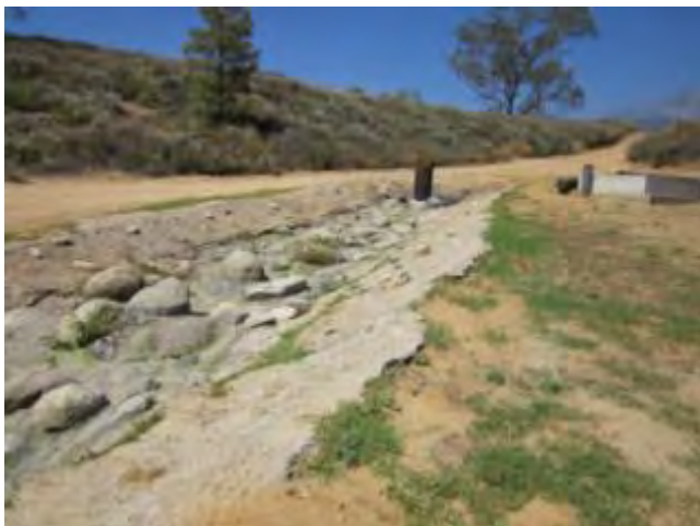
Water enters the park through a pipe and channel.
