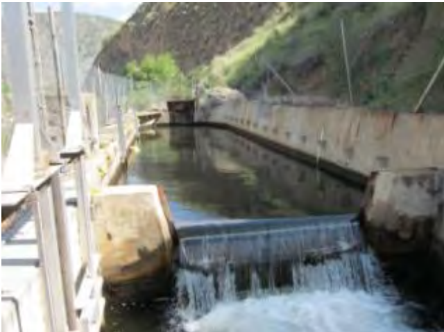
This weir measures the SAR water going to BVMWC.
