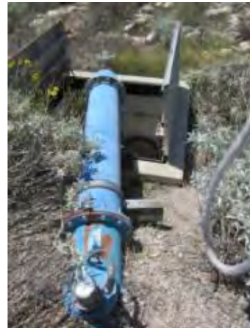
Gage can be used to verify SCADA's readings.
