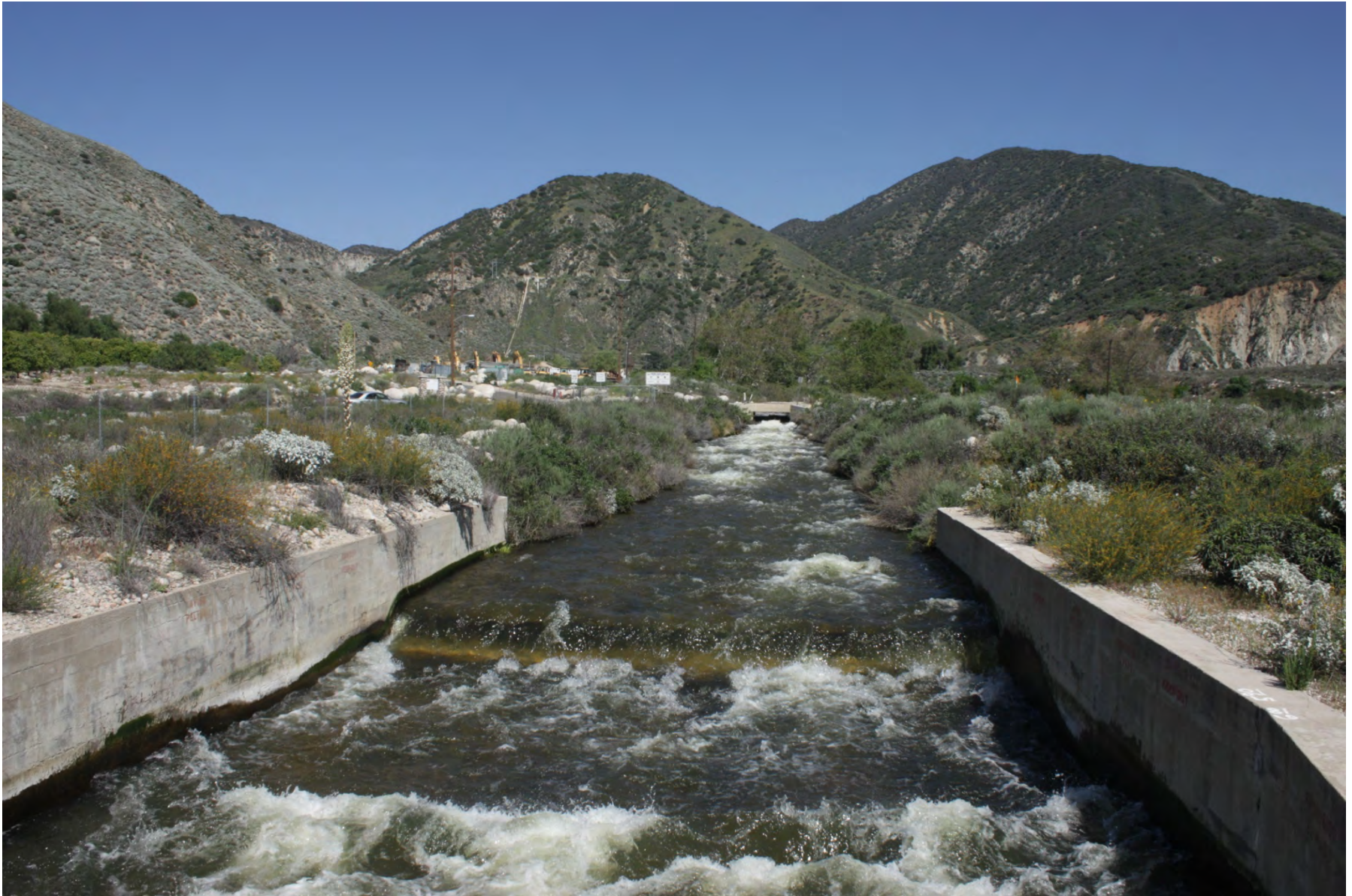
After passing through the District's intakes and under the Greenspot Road (located straight ahead), river flows enter this channel on their way to Basin 1. Photograph by Mathew O'Carroll.
