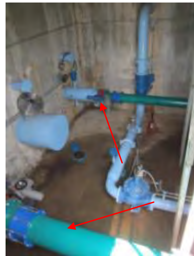
There is a high turnout and a low turnout (red arrows).
