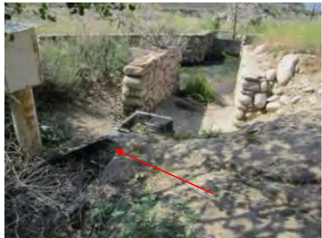
Water sent for spreading is measured at the Parshall Flume.
