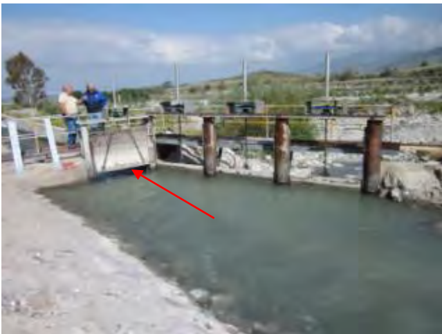
This gate allows MC water to enter diversion structure.
