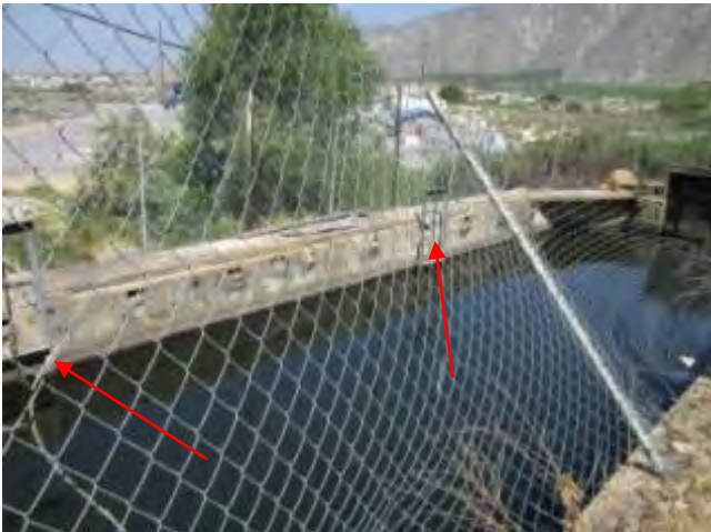
Water spills from sandbox through these 2 gates (red arrow).
