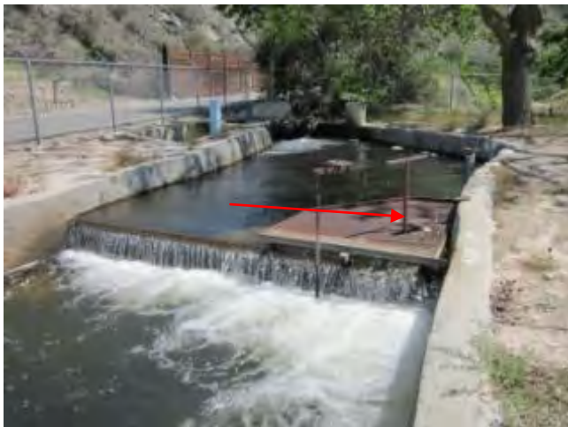
Water can be diverted at red arrow from NF Box to spreading.
