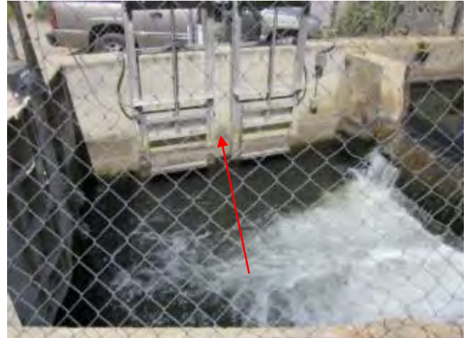
State Water enters the Sandbox through these gates (red arrow).
