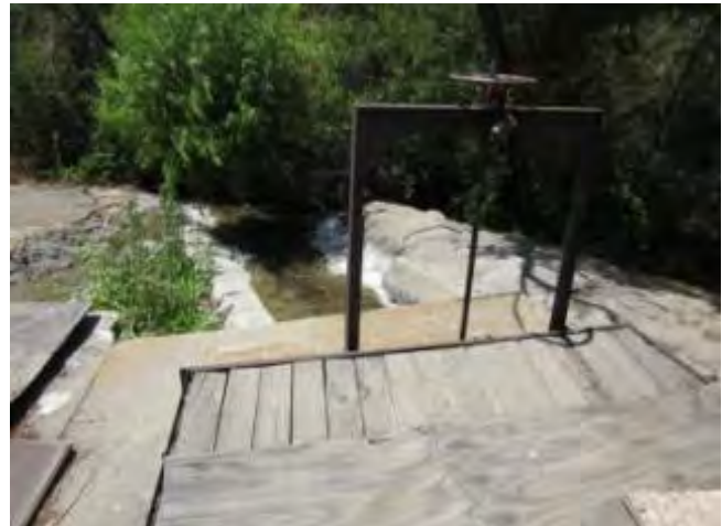
This sluice gate is opened to send water to Mill Creek.
