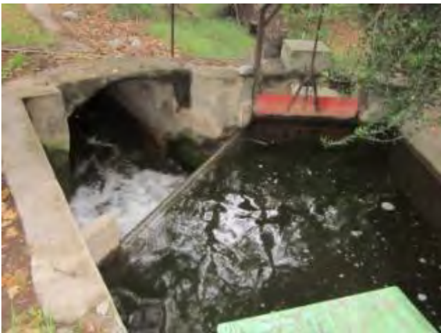
Left weir to Gay Overflow, Right Gate to Zanja
