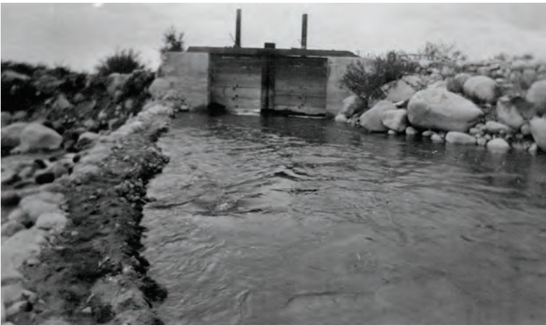
These were the first water gates installed by the Water Conservation Association, which was founded in 1909. Even now, simple cost-effective solutions often generate the highest returns.
