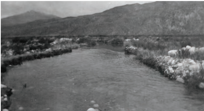
This is one of the earliest spreading grounds created by the Water Conservation Association. Floodwater from the Santa Ana River was spread across the ground where it then percolated to replenish the aquifer and provide a reliable source of well water.
